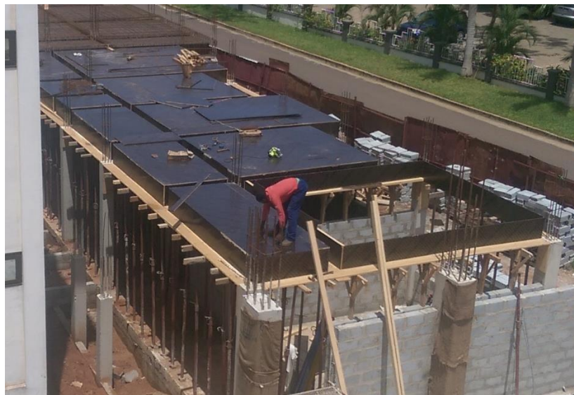
Progress of work on the WACCBIP building
